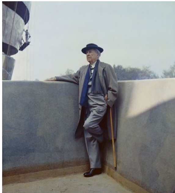
A dapper Frank Lloyd Wright poses on the balcony of the Solomon R. Guggenheim Museum during construction in 1959. Photo by William H. Short; from the Solomon R. Guggenheim Museum Archives
